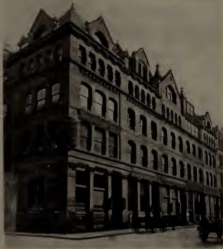
BUILDING, 60 to 78 Pearl Street, corner of Wendell. W. B. P. Weeks, Agent.
